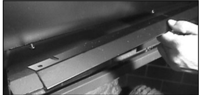
Figure 14.11 Installing the Hood
